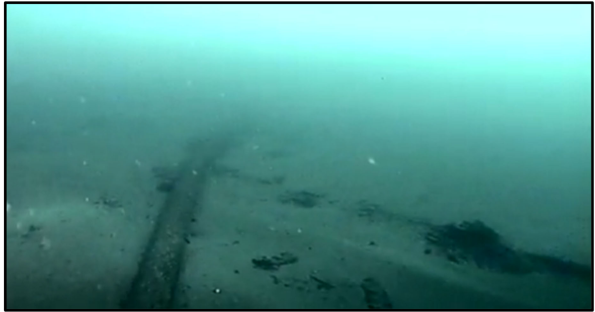
Image 9. Movement of Pipeline
